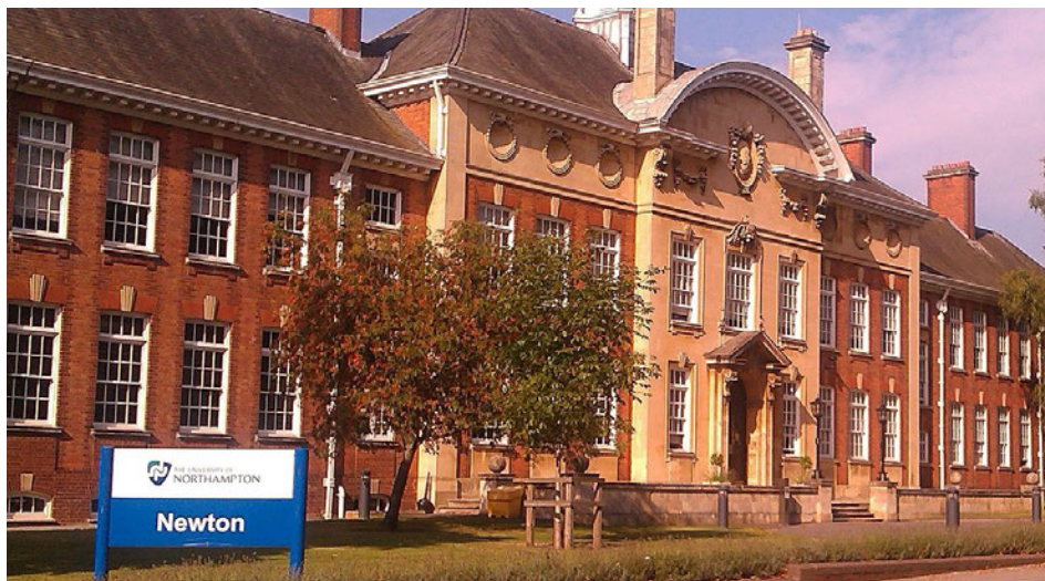
The School of Science and Technology, Newton Building, University of Northampton
